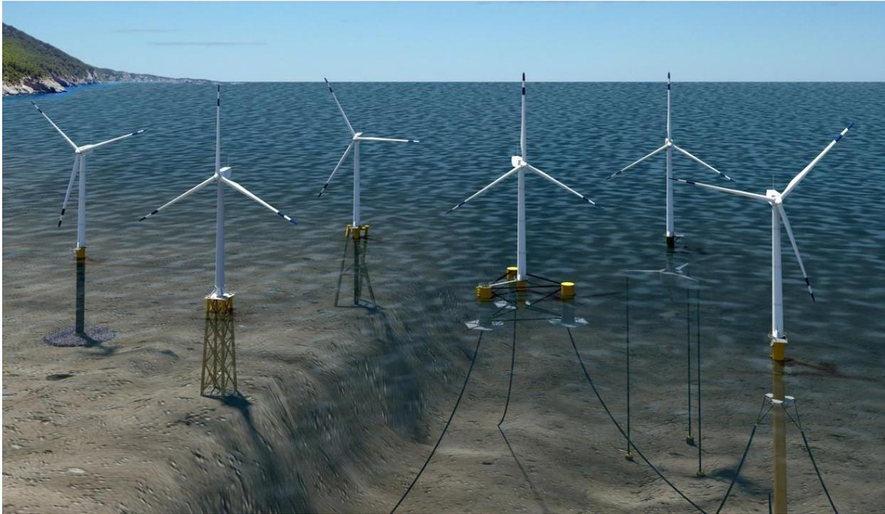
**Figure 1: Offshore wind foundation types**
